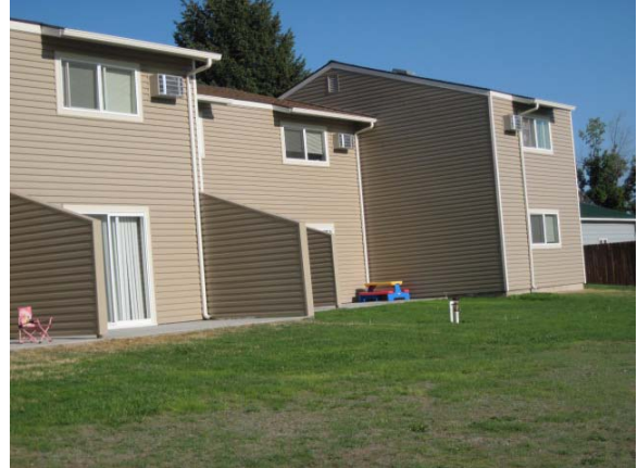
Back of Building D
