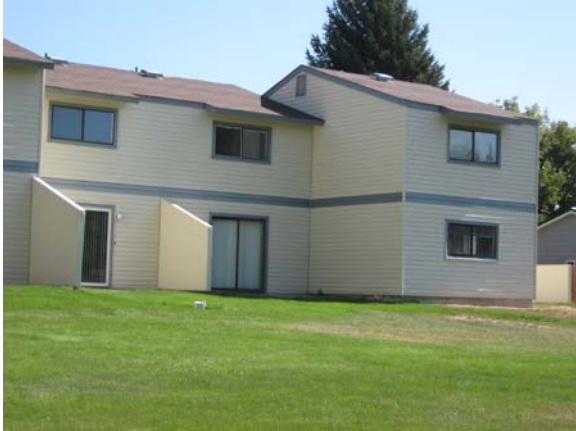
Back of Building D
