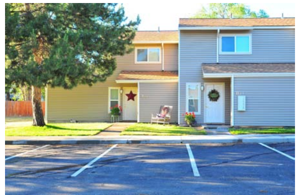
Front of Building B
