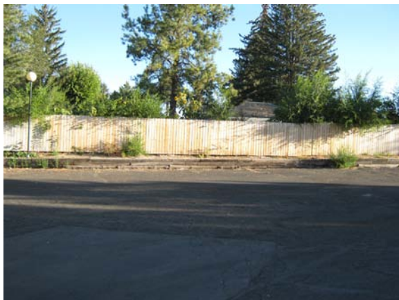
Railroad Tie Retaining Wall
