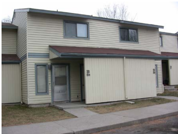
Front of Building B
