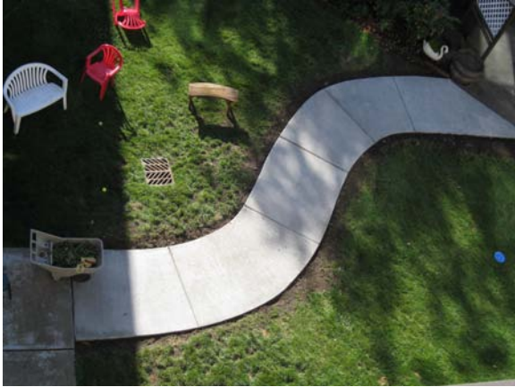
New concrete walkway
