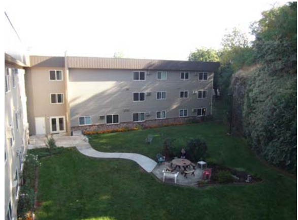
Side of Building after Walkway
