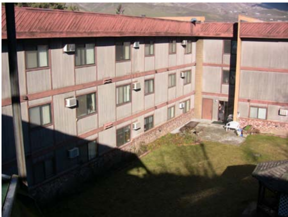
Side of Building before Walkway
