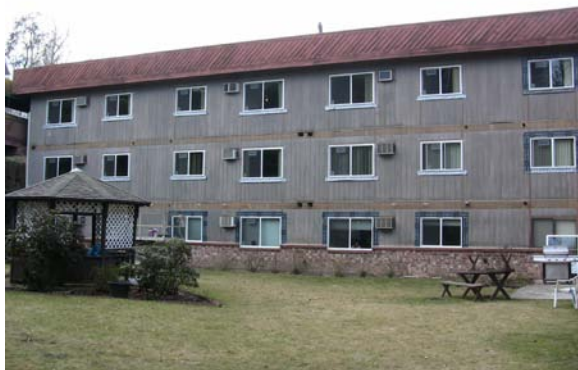
Side of Building with Gazebo
